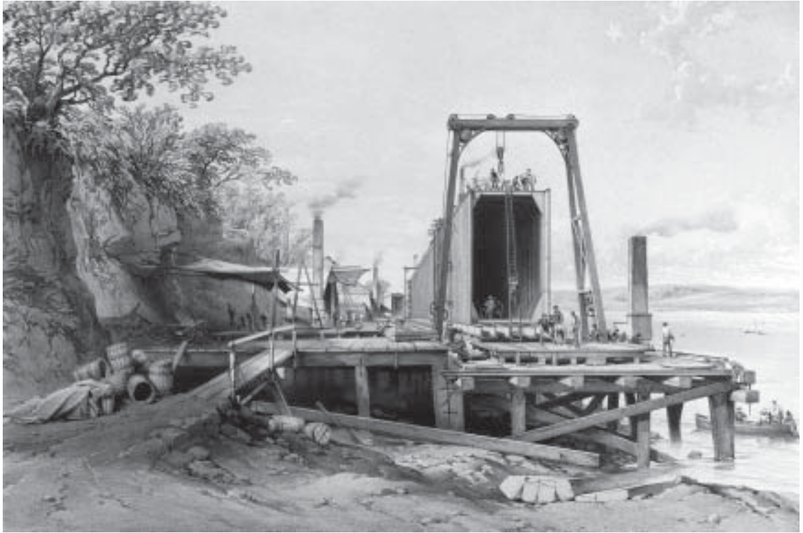
Detail of a tube under construction for the Britannia Bridge, from CLARK, E. The Britannia and Conway Tubular Bridges. London, 1850.
